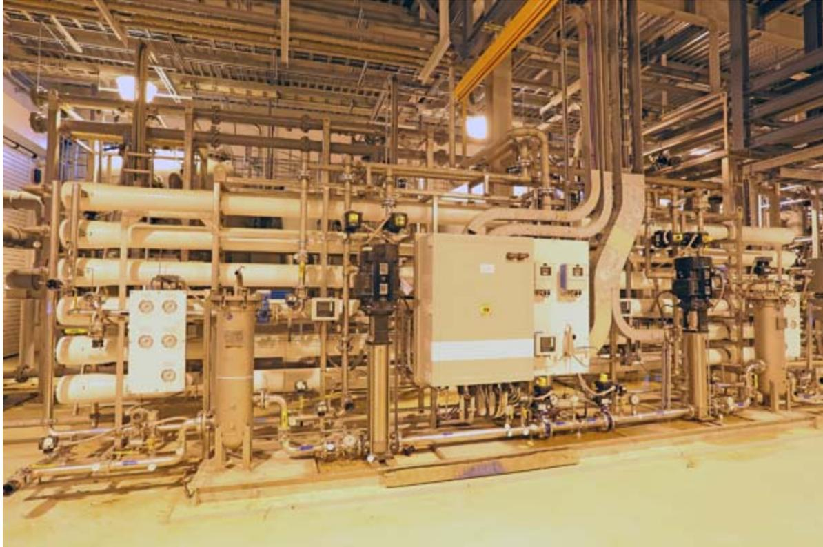
Figure 8 The RO pressure vessels in this industrial water system are placed horizontally, and vertically-oriented stainless steel pre-filter housings are in the foreground.
